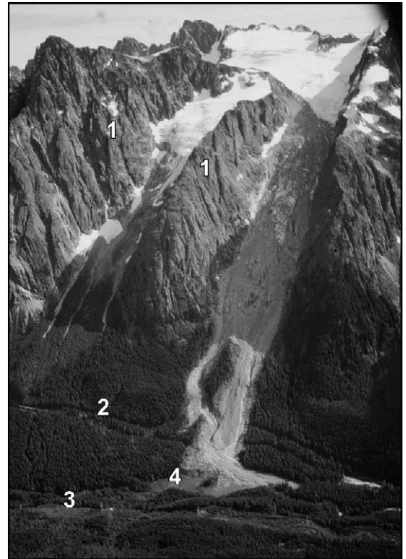
Fig. 4. Howson rock avalanche. Note cliffs (1), pipeline (2), powerline (3), and new lake (4).
